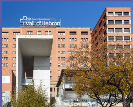
Hospital Val d'Hebrón, Barcelona, Spain
